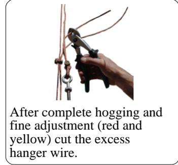
After complete hogging and fine adjustment (red and yellow) cut the excess hanger wire.
